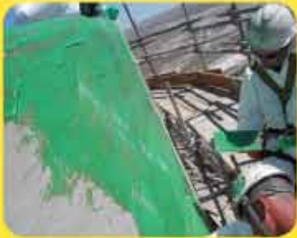
Application of tack coat
