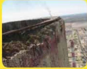
Significant decay and corrosion of concrete near the top of chimney
