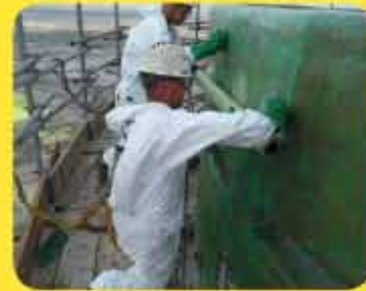
Installation of fabric
