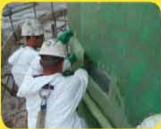
Installation of fabric
