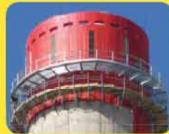
Restored chimney after repairs and painting
