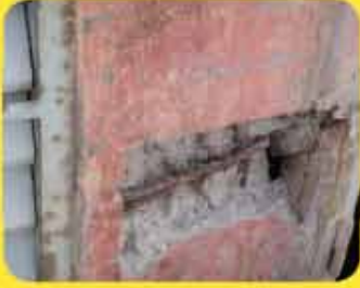
Significant decay and corrosion of concrete near the top of chimney
