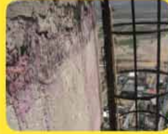
Significant decay and corrosion of concrete near the top of chimney
