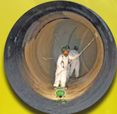
Top coating of CFRP in a curved, large-diameter PCCP
