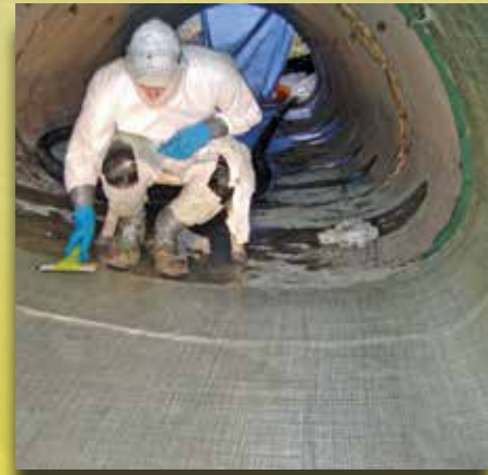
Repair of joints in oval-shaped concrete culvert
