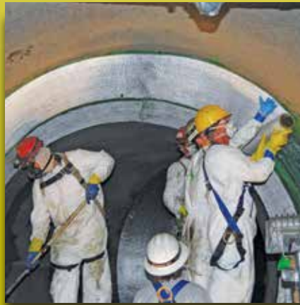
Glass fabric applied as dielectric barrier on steel pipe
