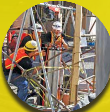
Equipment is delivered through access ports to avoid open cut trenches
