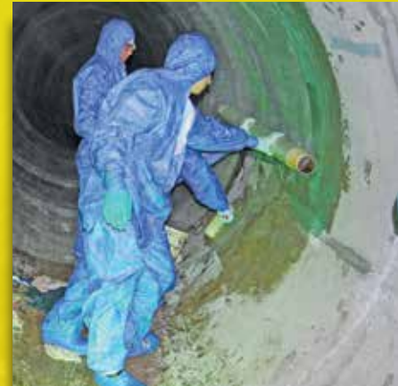
Applying pre-saturated roll of fabric to concrete pipe
