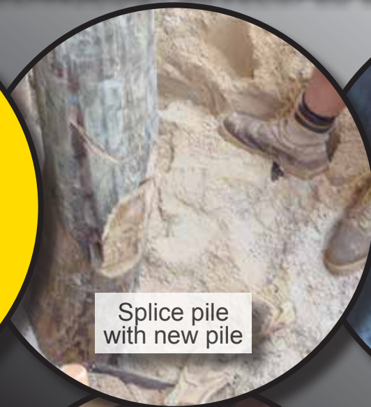
Place carbon strips around splice
