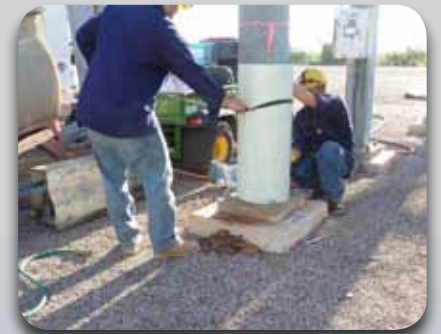
Use ratchet straps to support shell temporarily
