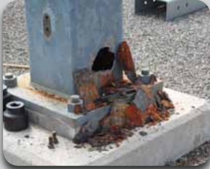
Corrosion-damaged column
