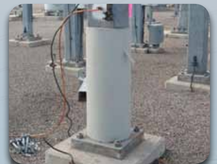
Remove ratchet straps & paint jacket (if desired)
