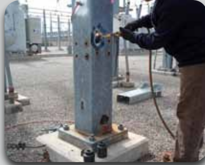
Cut an opening at 30-inch above grade
