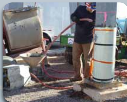
Fill the annular space with grout & vibrate
